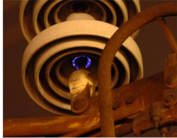
Streamer Corona in bottom of Insulator
